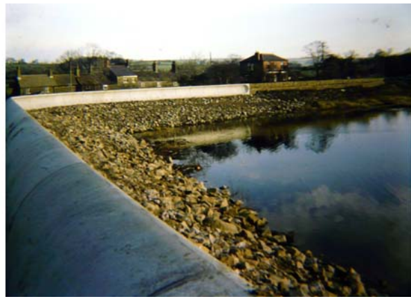
Installing a new wave wall on the dam – July and November 1983
