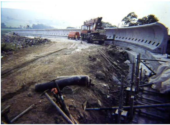
Installing a new wave wall on the dam – July and November 1983
